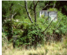
1 cassilis gold treatment works substation db
