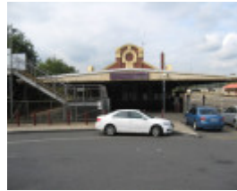
Warragul Railway Station entrance west end
