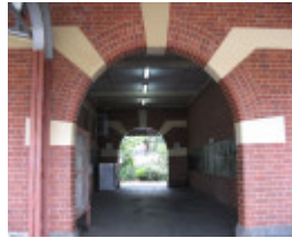
Warragul Railway Station link between 2 platforms
