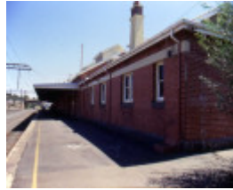
Warragul Railway Station
