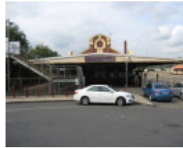
Warragul Railway Station entrance west end
