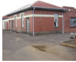
Warragul Railway Station drivers room
