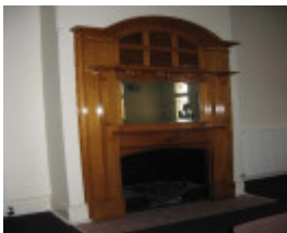
Warragul Railway Station fireplace in former dining room
