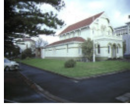
1 warrnambool court house gillies street warrnambool front view jan1983
