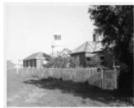
h01520 lady bay lighthouse complex 1962
