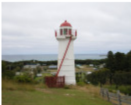
LADY BAY LIGHTHOUSE COMPLEX SOHE 2008
