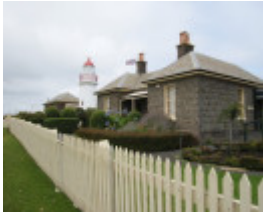
LADY BAY LIGHTHOUSE COMPLEX SOHE 2008
