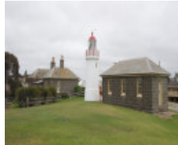
LADY BAY LIGHTHOUSE COMPLEX SOHE 2008
