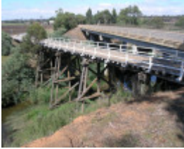
TRESTLE BRIDGE SOHE 2008
