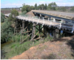
TRESTLE BRIDGE SOHE 2008
