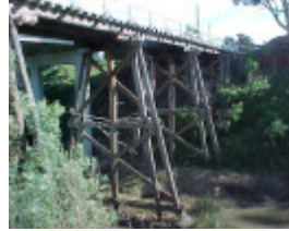
1 trestle bridge toward new bridge may01
