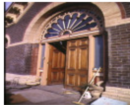
former albert park railway station complex ferrars street albert park front entrance jun1998
