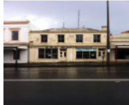
Appearance prior to repairs in 2013
