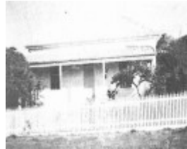
13 Flinders Street, Queenscliff
