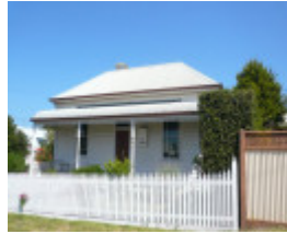
13 Flinders Street, Queenscliff
