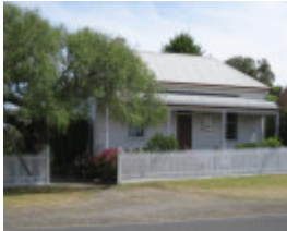
13 Flinders Street, Queenscliff
