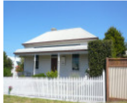
13 Flinders Street, Queenscliff
