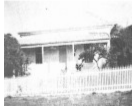
13 Flinders Street, Queenscliff
