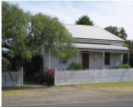
13 Flinders Street, Queenscliff
