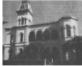
Lathamstowe, 44 Gellibrand Street, Queenscliff
