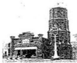
East Ballarat Fire Station - Ballarat Conservation Study, 1978
