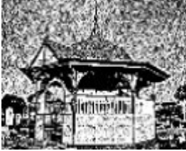
Centre Avenue Pavilion - Ballarat Heritage Review, 1998
