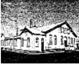
Drill Hall Curtis St - Ballarat Heritage Review, 1998
