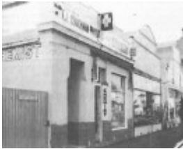
Former Bank of Victoria, 76 Hesse Street, Queenscliff
