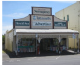
Former Bank of Victoria, 76 Hesse Street, Queenscliff
