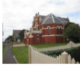
St Andrews Uniting Church and church hall
