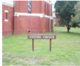
St Andrews Uniting Church and church hall
