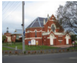
St Andrews Uniting Church and church hall
