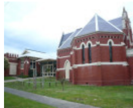
St Andrews Uniting Church and church hall
