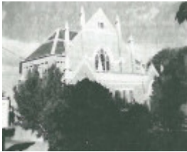
St Andrews Uniting Church, 83-89 Hesse Street
