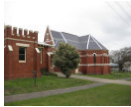
St Andrews Uniting Church and church hall
