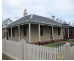
St Andrews Uniting Church and church hall
