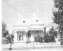
Carnbrea, 95 Hesse Street, Queenscliff
