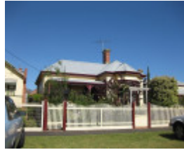
Romford, 105 Hesse Street, Queenscliff
