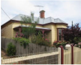
Romford, 105 Hesse Street, Queenscliff
