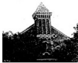
Lutheran Church Doveton St South - Film 9 / Frame 4 - Ballarat Conservation Study, 1978
