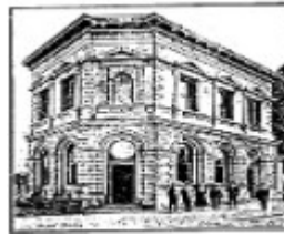
former gas company - Early photograph from Ballarat Illustrated - Ballarat Conservation Study, 1978
