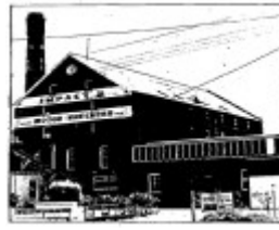
Former Myer Woollen Mill - Ballarat Conservation Study, 1978
