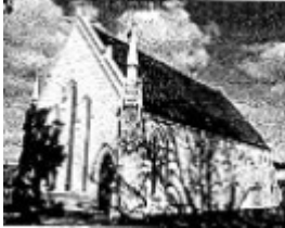
Uniting Church Brown Hill - Ballarat Heritage Review, 1998
