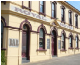
Royal Hotel, 34-38 King Street, Queenscliff
