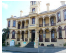
Royal Hotel, 34-38 King Street, Queenscliff
