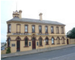
Royal Hotel, 34-38 King Street, Queenscliff
