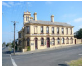
Royal Hotel, 34-38 King Street, Queenscliff
