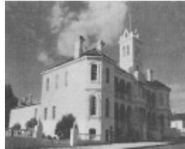
Royal Hotel, 34-38 King Street, Queenscliff
