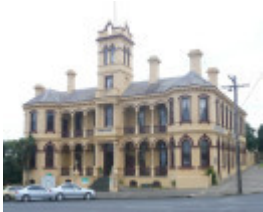
Royal Hotel, 34-38 King Street, Queenscliff
