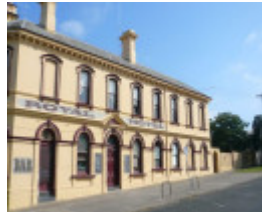
Royal Hotel, 34-38 King Street, Queenscliff
