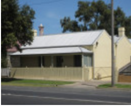
39 King Street, Queenscliff
