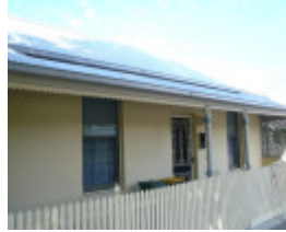
39 King Street, Queenscliff
