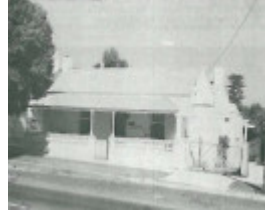
39 King Street, Queenscliff
