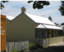
39 King Street, Queenscliff
