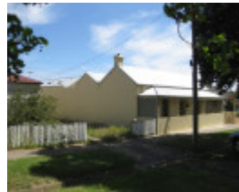
39 King Street, Queenscliff
