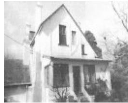
Former St. Georges Church of England Parsonage, 13 Mercer Street, Queenscliff
