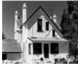
Former St George's Church Vicarage c. 1972-1983 Source: Pictures Collection, State Library of Victoria
