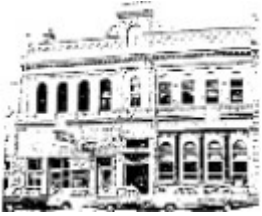
Booths Buildings - Film 1 / Frame 36 - Ballarat Conservation Study, 1978
