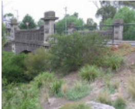
BRIDGE OVER MOONEE PONDS CREEK SOHE 2008
