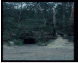
FOURTH HILL TUNNEL
