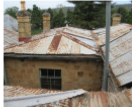
121693_former survey office_Helenslee_Heathcote_A (1).jpg
