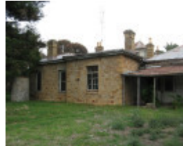
121693_former survey office_Helenslee_Heathcote_A (1).jpg
