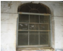
121693_former survey office_Helenslee_Heathcote_A (1).jpg
