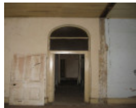
121693_former survey office_Helenslee_Heathcote_A (1).jpg
