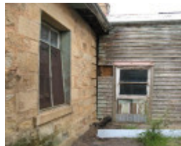
121693_former survey office_Helenslee_Heathcote_A (1).jpg
