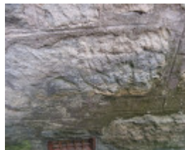
121693_former survey office_Helenslee_Heathcote_A (1).jpg
