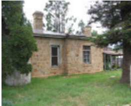
121693_former survey office_Helenslee_Heathcote_A (10).jpg
