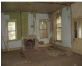
121693_former survey office_Helenslee_Heathcote_A (1).jpg
