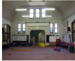
h01639 primary school no 1183 cnr cecil and parker street williamstown interior she project 2004
