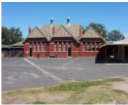
h01639 primary school no 1183 cnr cecil and parker street williamstown side view she project 2004
