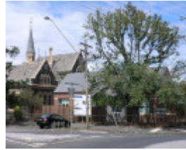
WILLIAMSTOWN PRIMARY SCHOOL NO. 1183 SOHE 2008
