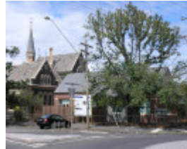
WILLIAMSTOWN PRIMARY SCHOOL NO. 1183 SOHE 2008
