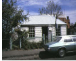
1 residence 11 cox's gardens williamstown front view oct1980
