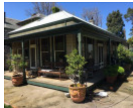
Northwest corner of mid-1980s single-storey addition.
