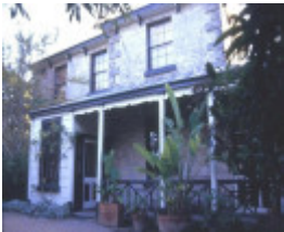
h00229 former presbyterian manse lyons st williamstown close up she project 2003
