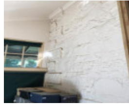
Within enclosed north verandah, looking at painted stone wall at northeast corner of Former Manse
