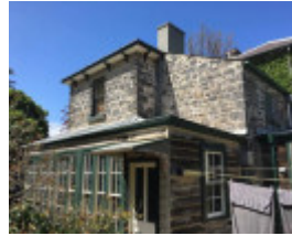
Northwest corner of bluestone fabric, showing two-storey skillion-roof portion, with the enclosed timber-framed verandah of the north elevation in foreground.
