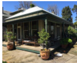
Northwest corner of mid-1980s single-storey addition.
