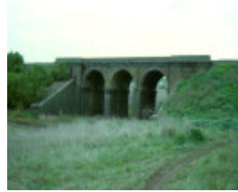
H01964 sunbury rail bridge
