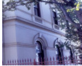
former customs house cnr nelson place and syme st williamstown close up windows she project 2003
