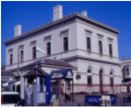
former customs house cnr nelson place and syme st williamstown cnr view she project 2003
