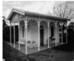
anne caudle centre entrance gatehouse
