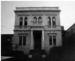
1 anne caudle centre front view superintendents building
