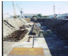
h00697 alfred graving dock williamstown dockyard williamstown front view
