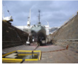
ALFRED GRAVING DOCK SOHE 2008
