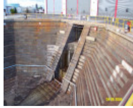
h00697 alfred graving dock williamstown dockyard williamstown steps she project 2004
