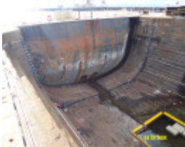
h00697 alfred graving dock williamstown dockyard williamstown close up she project
