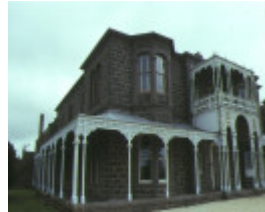
1 barwon park inverleigh rd winchelsea front view homestead
