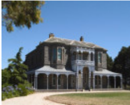
H0365 BARWON PARK - National Trust of Australia (Vic)
