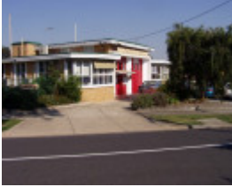
Rosanna Metropolitan Fire Brigade Station
