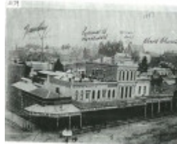
Union Hotel in 1887 showing additional floor
