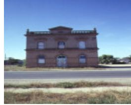
1 mechanics institute carlisle street wunghnu front view apr1981
