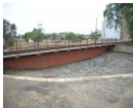
WYCHEPROOF RAILWAY STATION SOHE 2008
