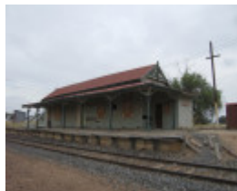
WYCHEPROOF RAILWAY STATION SOHE 2008
