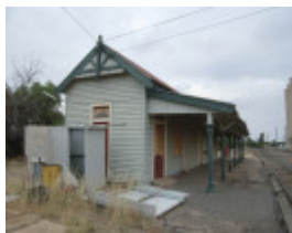
WYCHEPROOF RAILWAY STATION SOHE 2008
