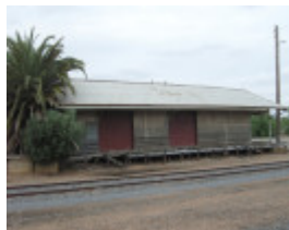
WYCHEPROOF RAILWAY STATION SOHE 2008
