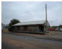
WYCHEPROOF RAILWAY STATION SOHE 2008
