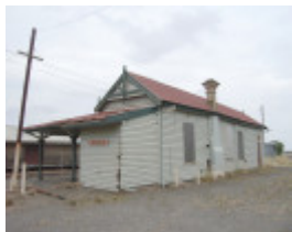
WYCHEPROOF RAILWAY STATION SOHE 2008
