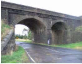
B 6394 Cowies Creek Bridge No. 1
