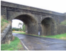
B 6394 Cowies Creek Bridge No. 1
