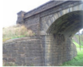
B6394 Cowies Creek Bridge No. 1 wall
