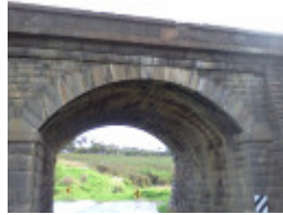
B6394 Cowies Creek Bridge No. 1 arch.
