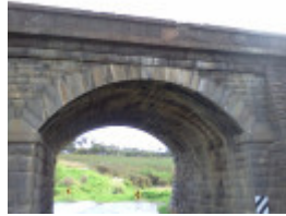
B6394 Cowies Creek Bridge No. 1 arch.
