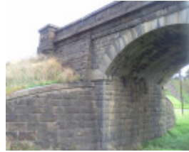
B6394 Cowies Creek Bridge No. 1 wall
