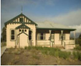
Former Shire Offices and Library, 60 Beverley Road
