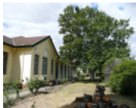
KYNETON SECONDARY COLLEGE (FORMER HIGH SCHOOL) SOHE 2008
