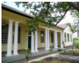
KYNETON SECONDARY COLLEGE (FORMER HIGH SCHOOL) SOHE 2008
