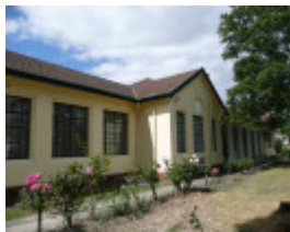
KYNETON SECONDARY COLLEGE (FORMER HIGH SCHOOL) SOHE 2008
