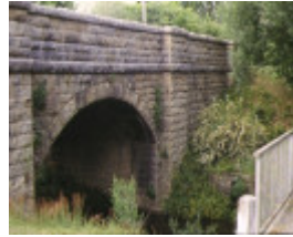
1 bridge over commissioners creek yackandandah side view
