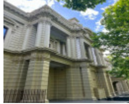
2023. Western facade, near Lyttleton Terrace
