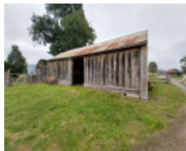
Vertical timber slab stables. 2023.
