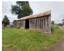
Vertical timber slab stables. 2023.
