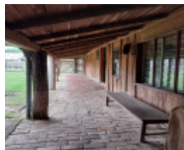
verandah to kitchen block, 2023.
