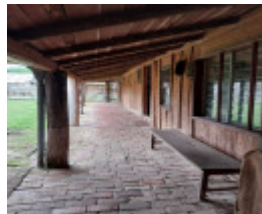
verandah to kitchen block, 2023.
