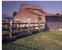
h00384 gulf station melba hwy yarraglen shearing shed west wall she project 2003
