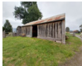
Vertical timber slab stables. 2023.
