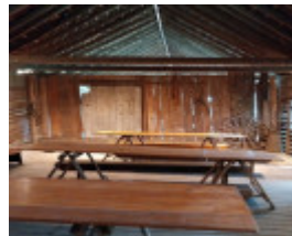
Shingle ceiling in the shed, 2023.
