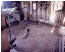
h00384 gulf station melba hwy yarraglen shearing shed interior she project 2003
