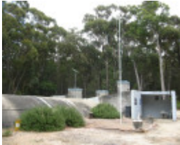
External view to the west, Feb 2008.
