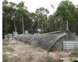
External view to the east, Feb 2008.
