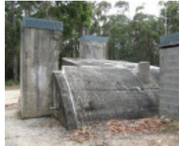
Western end, external view of engine room, Feb 2008.
