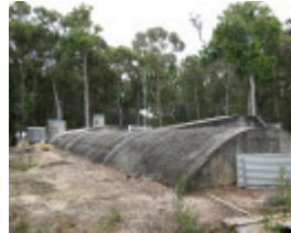
External view to the east, Feb 2008.
