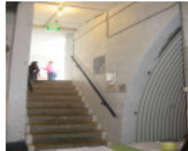
Internal view of west stair well, Feb 2008.
