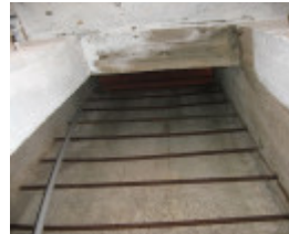
Looking up the escape hatch and air shaft at western end of building, Feb 2008.
