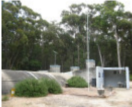
External view to the west, Feb 2008.
