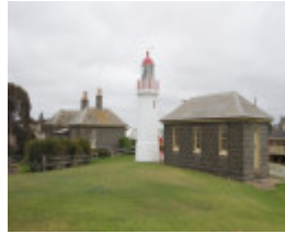
LADY BAY LIGHTHOUSE COMPLEX SOHE 2008
