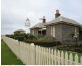
LADY BAY LIGHTHOUSE COMPLEX SOHE 2008
