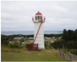
LADY BAY LIGHTHOUSE COMPLEX SOHE 2008
