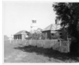
h01520 lady bay lighthouse complex 1962
