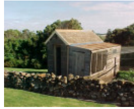
h01520 lady bay lighthouse complex privy jun04 pm1
