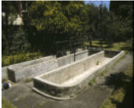
1 sicree family air raid shelter mitford street st kilda elevated view of shelter jan1995
