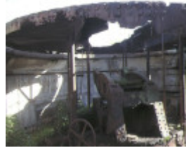
1 south channel fort gun emplacement jun1989
