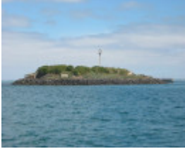
SOUTH CHANNEL FORT SOHE 2008
