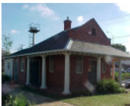
H01098 rafa barracks guard room 2001 pm1
