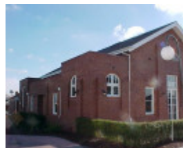
H01098 rafa barracks gymnasium 2001 pm1
